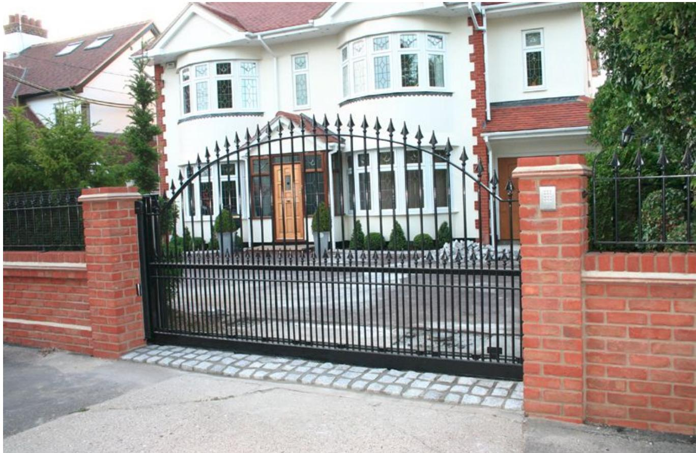
Sliding electric gates can come a track or trackless also known as a cantilever gate. When installing a tracked sliding gate it is important that the floor surface is level.
