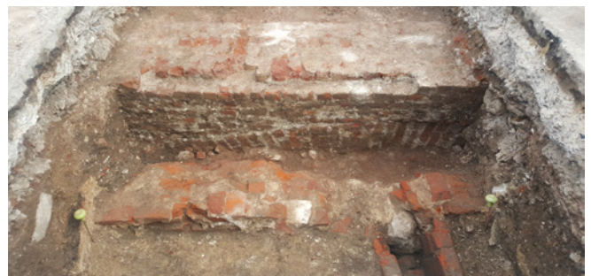
Brickwork recorded in this trial hole is thought to relate to the 16th/17th century Whitehall Palace, and has been retained in situ. Other underground constraints include utilities and tree roots.
