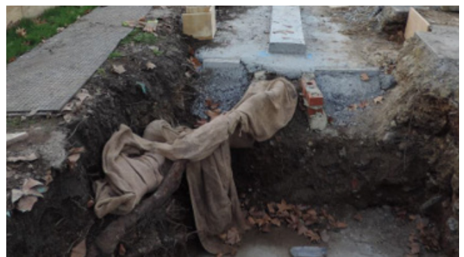
Brickwork recorded in this trial hole is thought to relate to the 16th/17th century Whitehall Palace, and has been retained in situ. Other underground constraints include utilities and tree roots.
