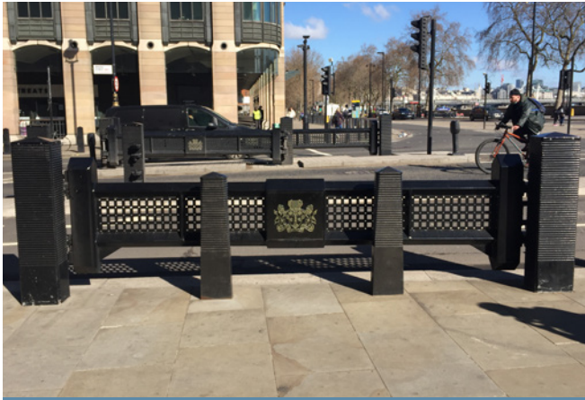
The alignment comprises four Westminster design gate types with gilded crests, in this wide highway location adjacent to the Houses of Parliament and integrated with footway improvements.
